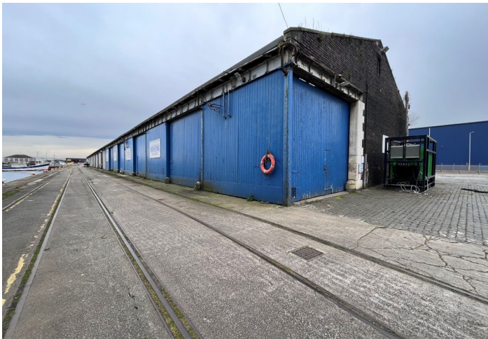
Edinburgh Dock Sheds
