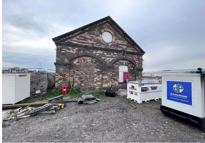
Listed Pumping House
