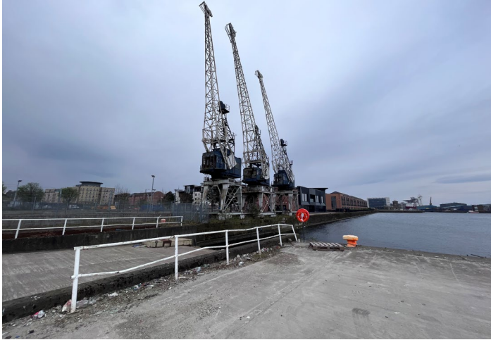
Looking North West Towards The Listed Cranes Fronting Albert Dock
