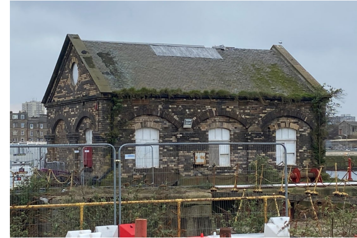
Listed Pumping House
