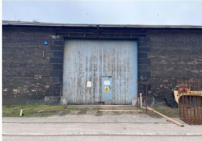
Edinburgh Dock Sheds
