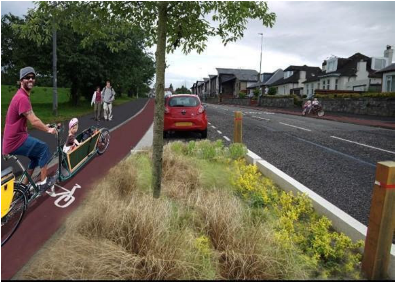
Image 3: floating parking with sustainable drainage, accessible kerbs and clearer parking spaces
