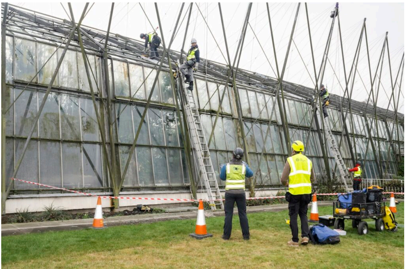
Glasshouse repairs underway in the Royal Botanic Garden
