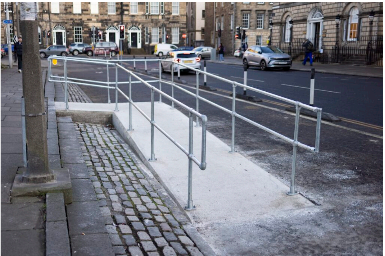
It is understood that the ramp is there to address accessibility concerns with the steps surrounding the square.
