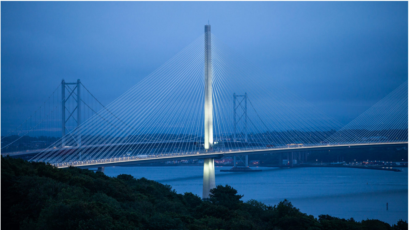
Queensferry Crossing Photo BEAR Scotland
