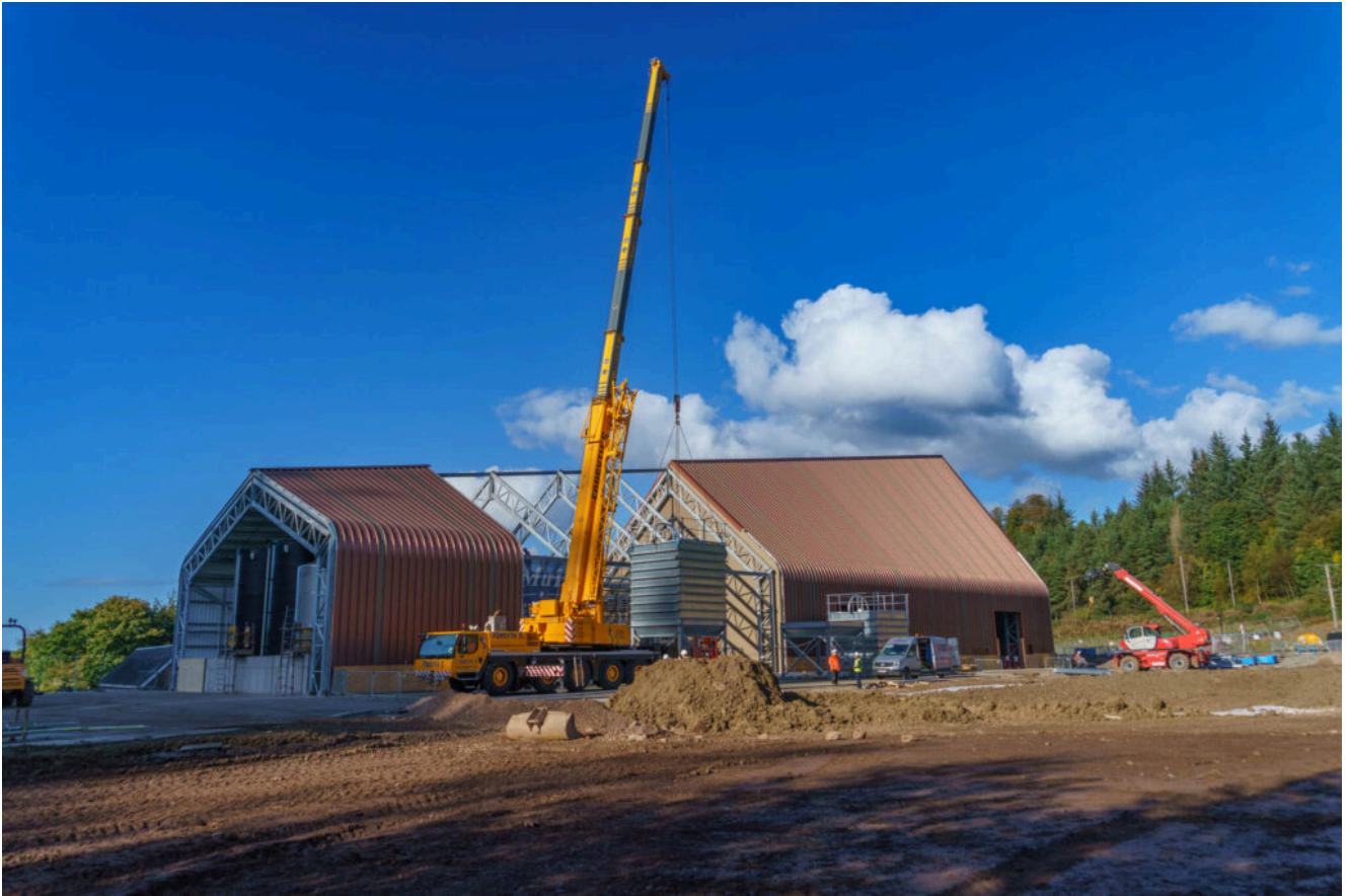
Ardgowan Distillery under construction at Bankfoot Farm Inverkip
