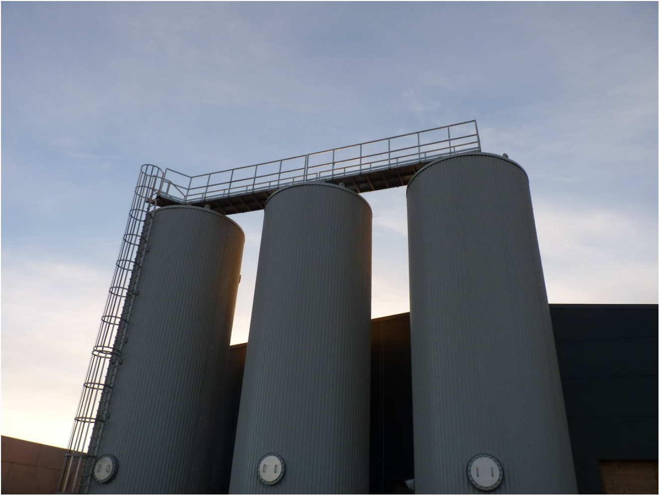
Midlothian Energy site is nearly ready to produce heating pic courtesy Vattenfall
