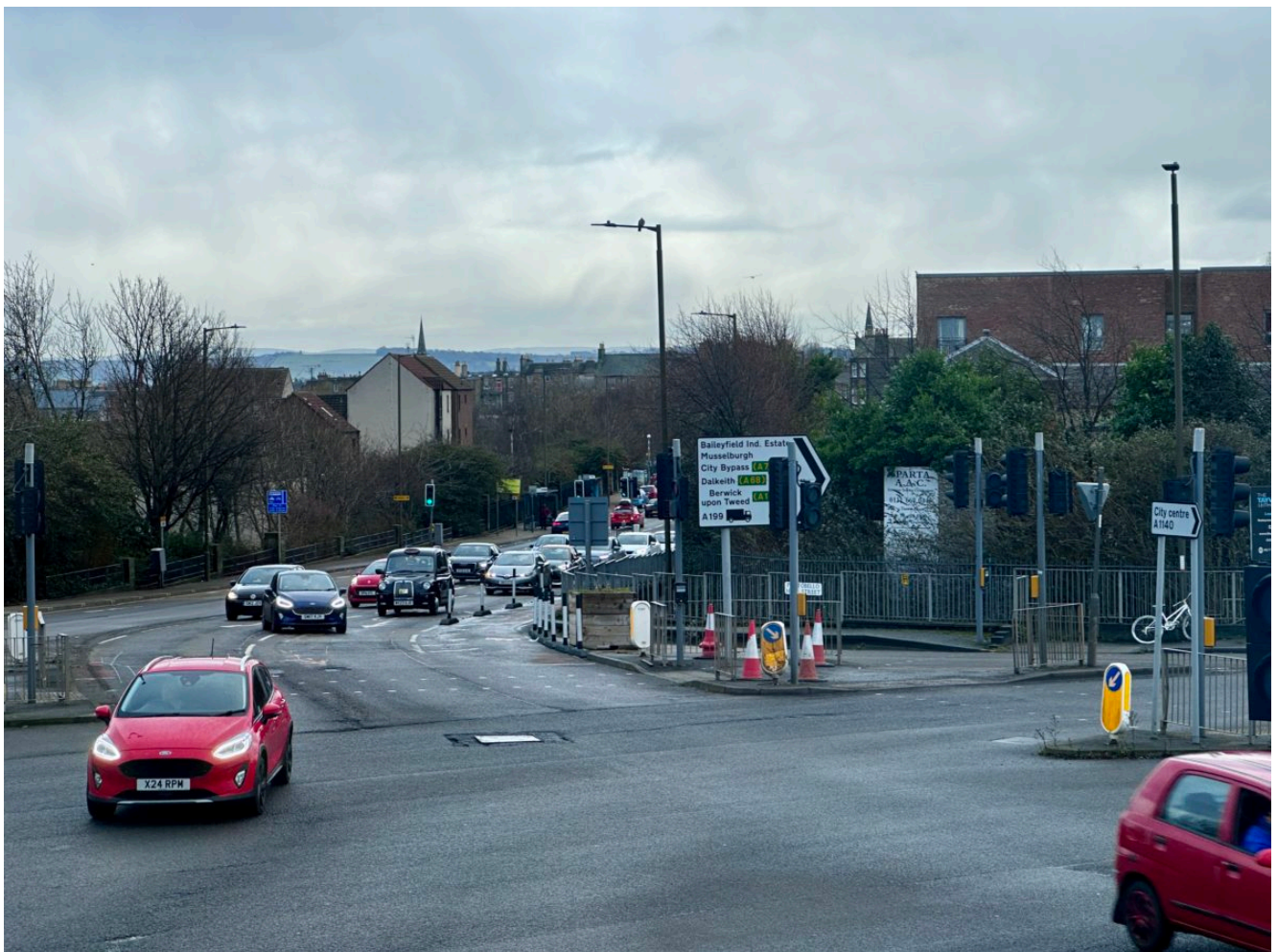
King's Road junction with Sir Harry Lauder Road where HGV traffic coming from Portobello can no longer turn left
