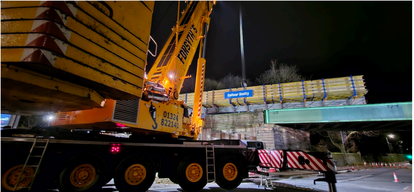
Dalry Road 21 November 2023 PHOTO Balfour Beatty
