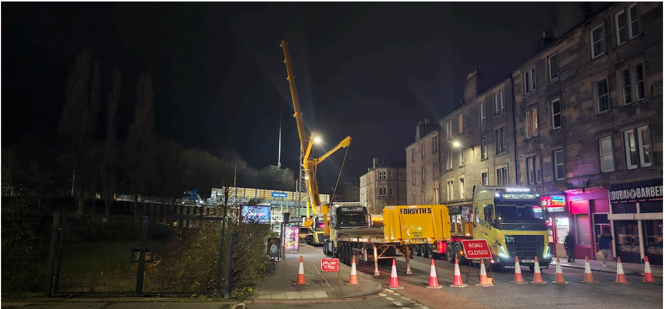
Dalry Road 21 November 2023 PHOTO Balfour Beatty
