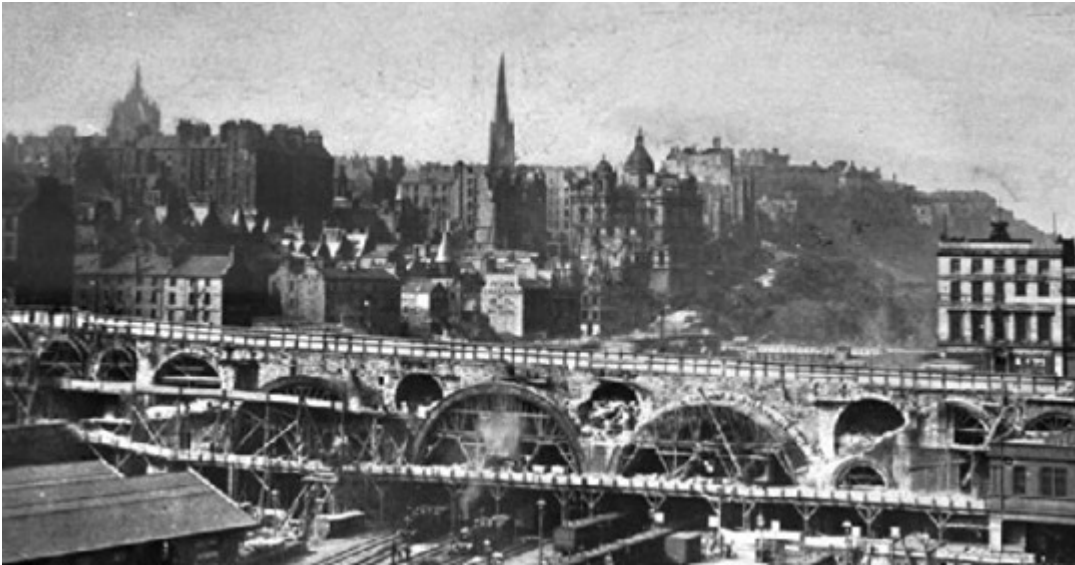
3 August Picture shows the original North Bridge during dismantling circa 1896
