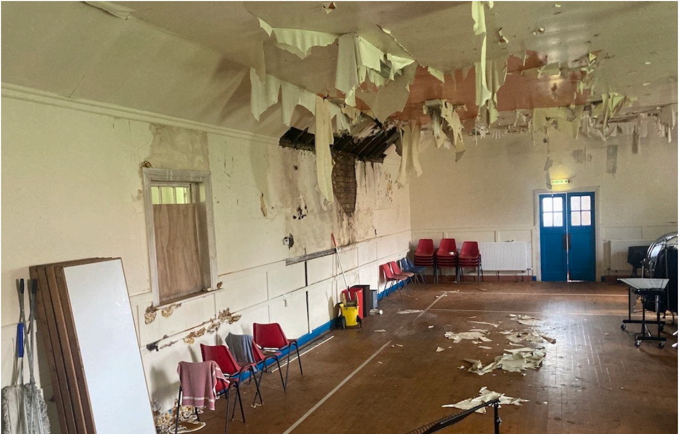
The main hall at Vogrie Hall with collapsed ceiling, leaking roof and fungus growing on walls. Pic staff
