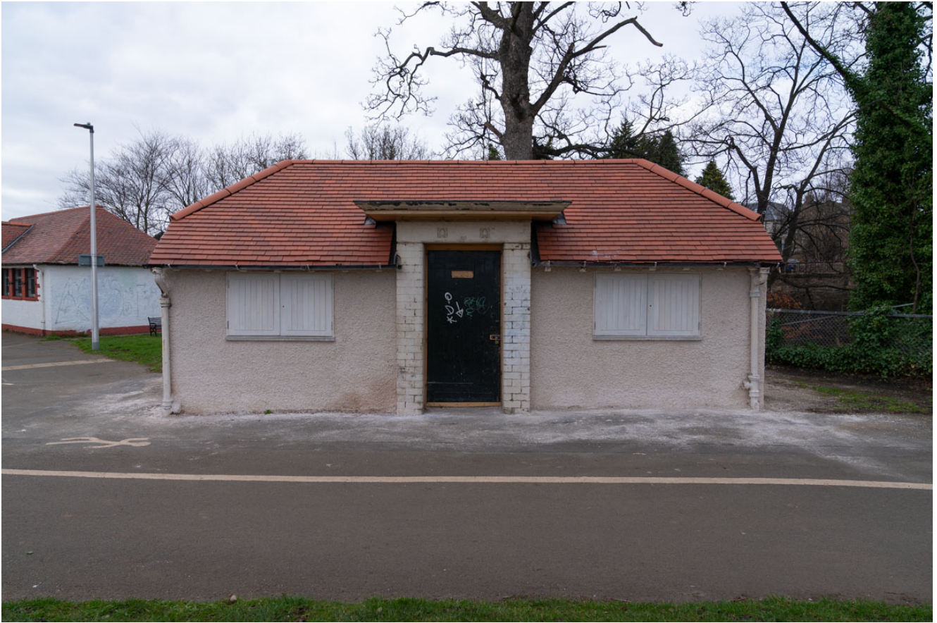
Roseburn – former toilets to become a café Photo © 2023 Martin P. McAdam www.martinmcadam.com
