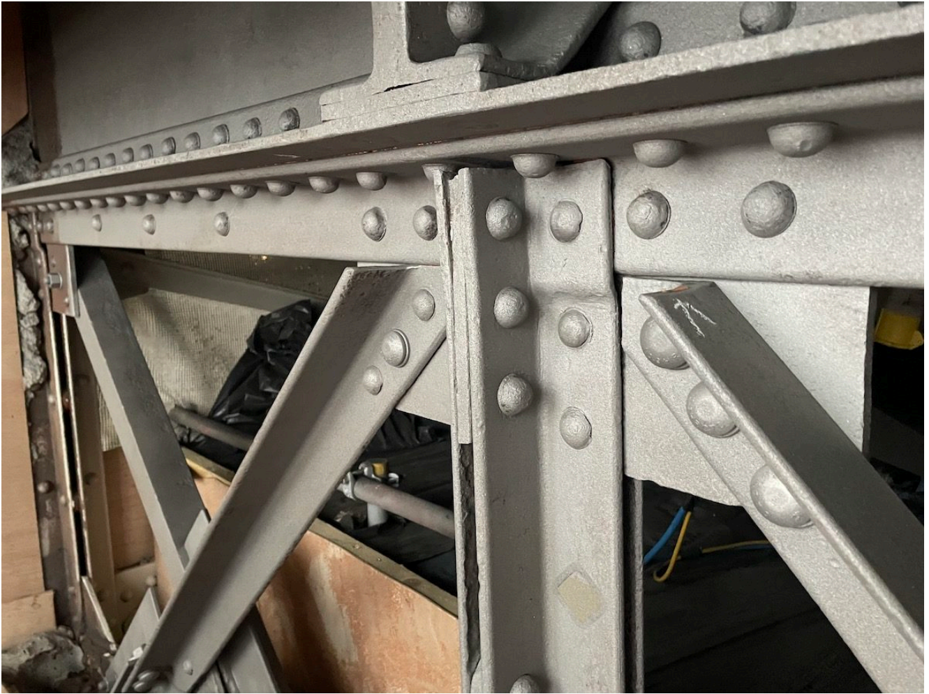
Freshly blasted 1890s steelwork
