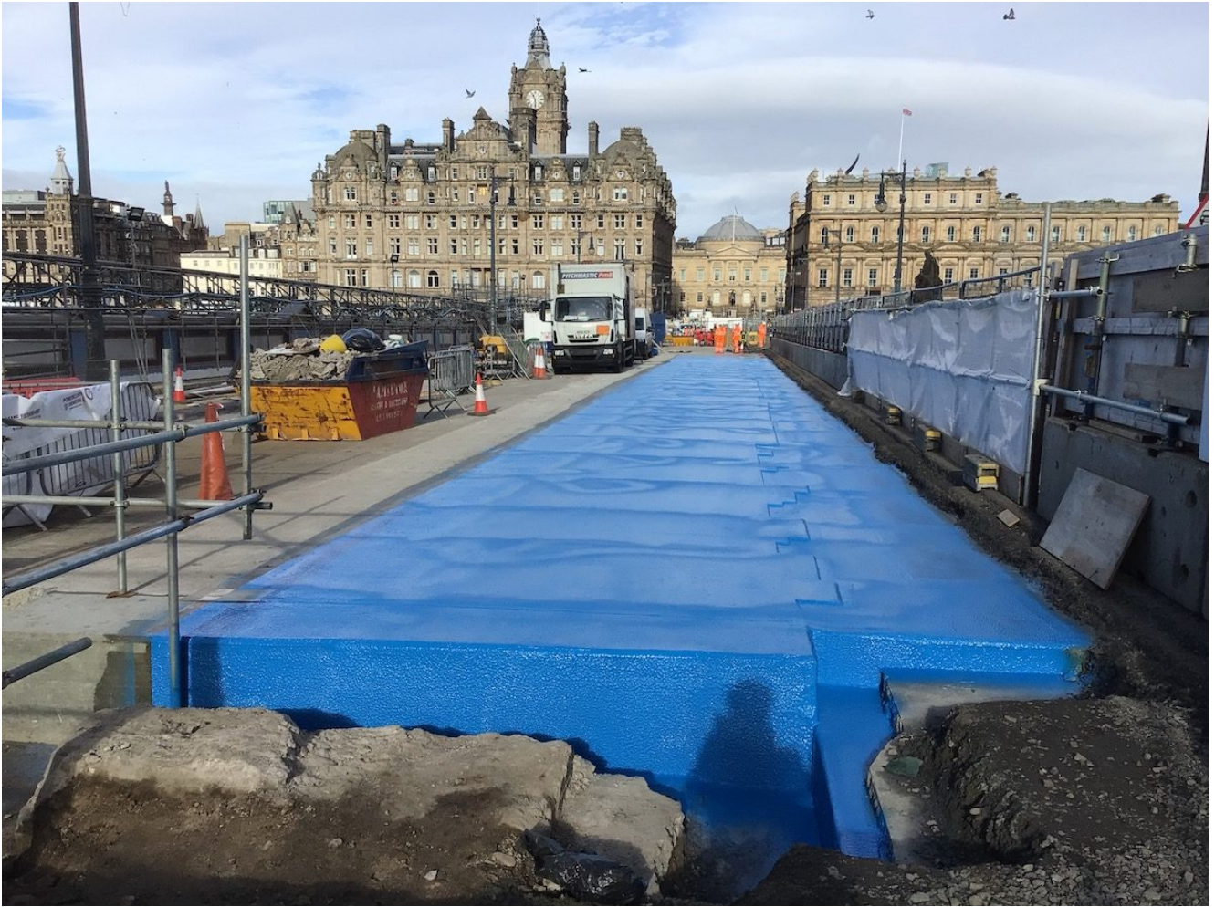
Waterproofing works
