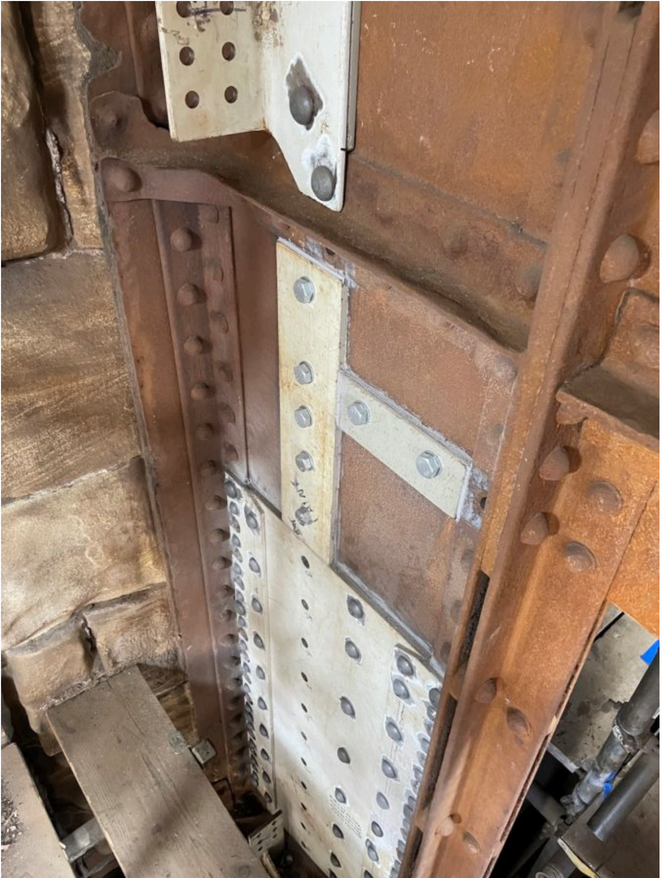
In progress steelwork repairs
