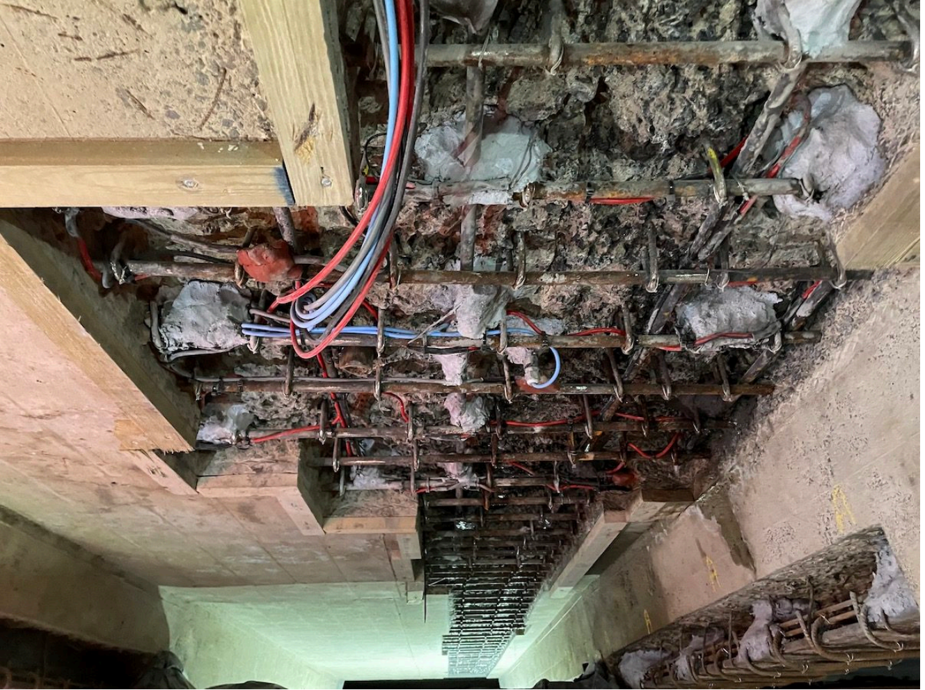
Concrete Deck Soffit Repairs
