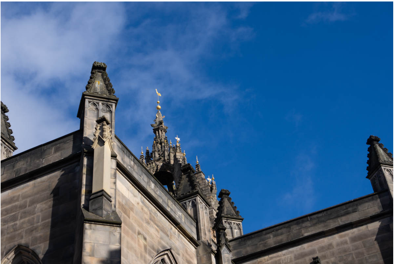
The roof at St Giles. ©2023 The Edinburgh Reporter
