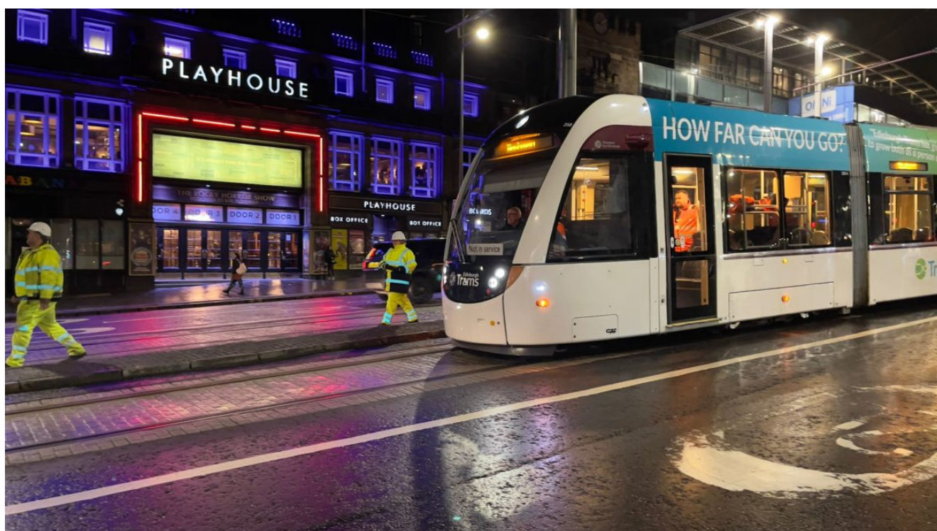
First trams since November 1956 go down Leith Walk on 13 March 2023 during testing phase PHOTO Thomas Haywood Photography
