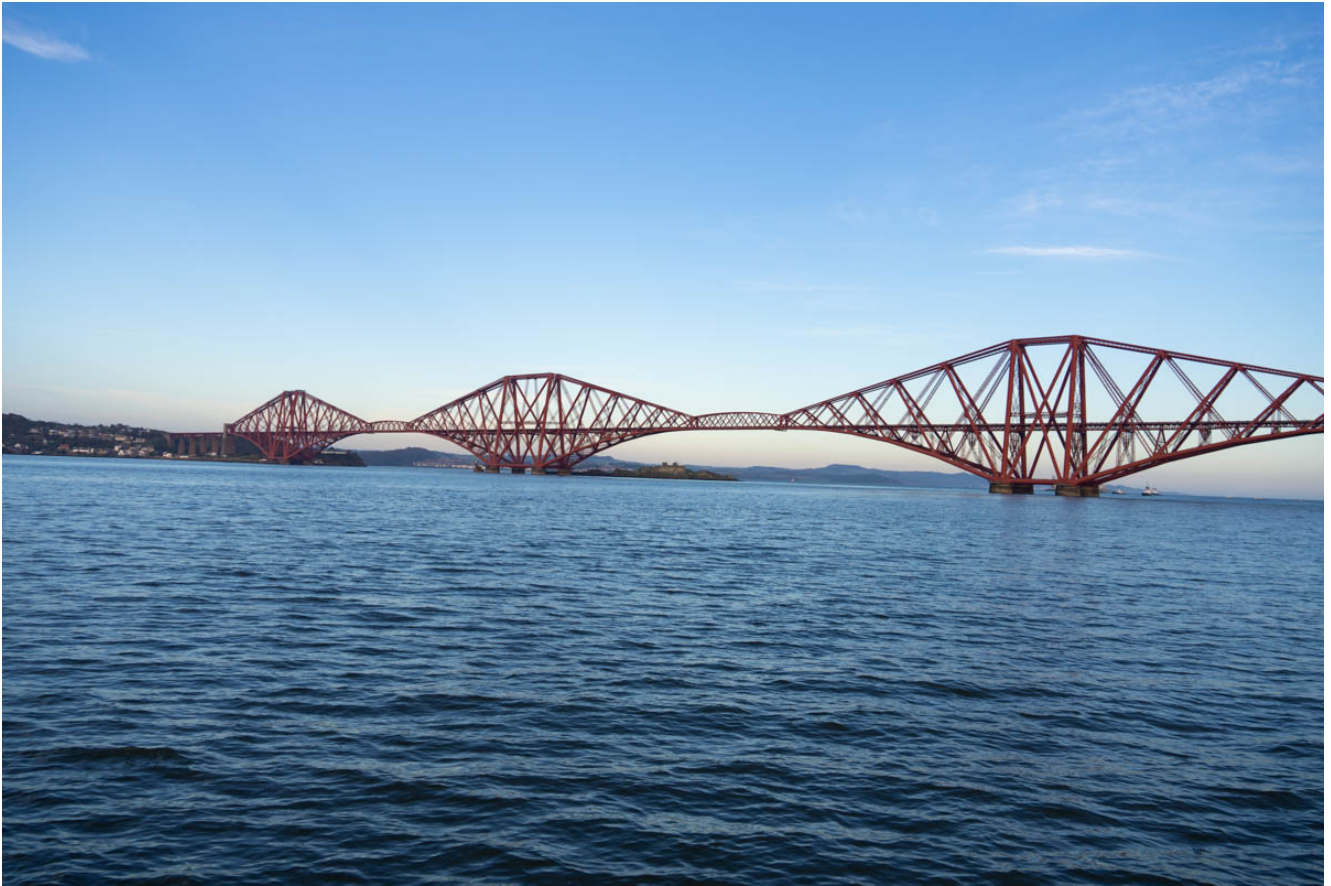
Forth Bridge PHOTO ©2022 The Edinburgh Reporter
