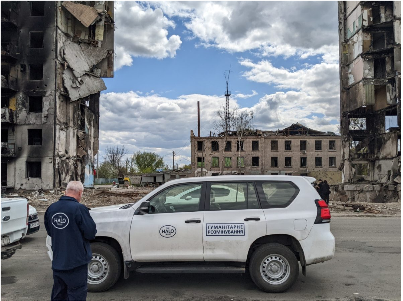
Survey work around Kyiv, May 2022
