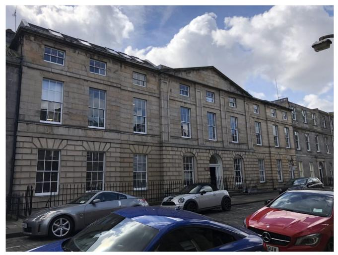
Modern Playfair House, fronting Broughton Street Lane, will be stripped back to its superstructure and a new facade of natural stone and precast concrete built to align with adjacent buildings, reinstating the mews street frontage, although Cllr Neil Rankin pointed out that the reuse was preferable to demolition.
