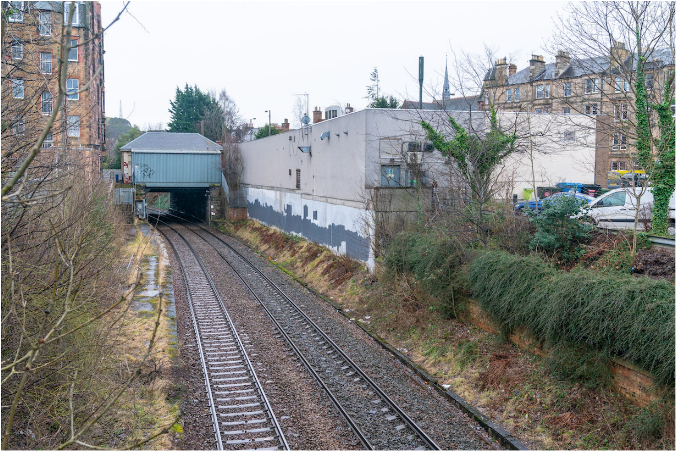
Morningside Station – the old platform. Photo: © 2021, Martin P. McAdam www.martinmcadam.com
