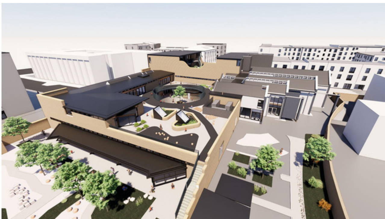
Aerial view from the west
