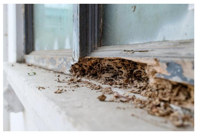
Termite damage on a wooden window frame. <u>Attapon</u> <u>Thana/Shutterstock</u>
