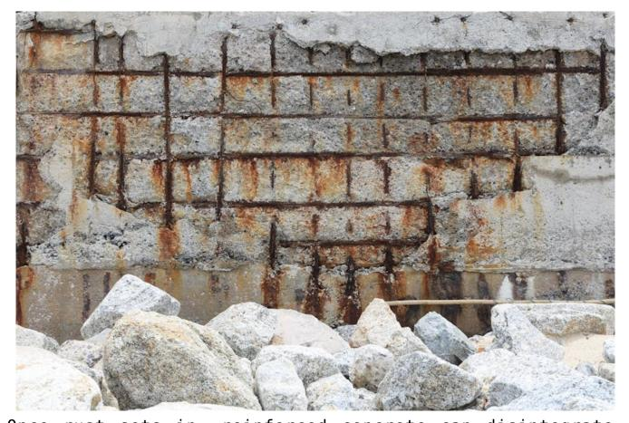
Once rust sets in, reinforced concrete can disintegrate. <u>Arayan Rattanaphan/Shutterstock</u> Buildings in coastal areas are especially susceptible as the chloride in salt water accelerates rusting. Rising sea levels will raise the water table and make it saltier, affecting building foundations, while salt-spray will spread further on stronger winds.
