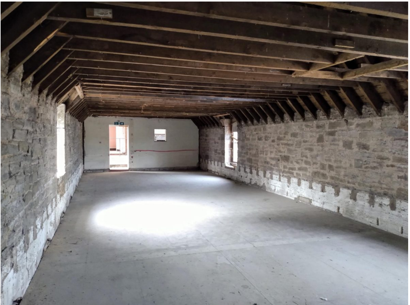
The interior of the stables in April 2021
