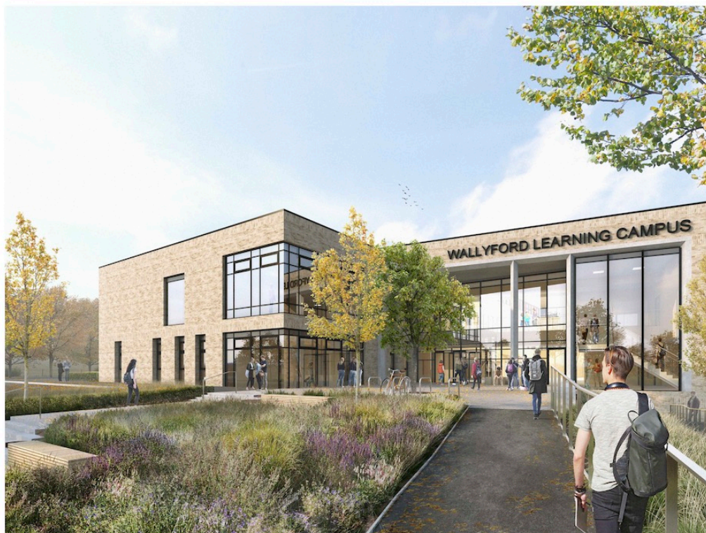
EXTERNAL VISUALISATION/01 View of east elevation towards Main Entrance
