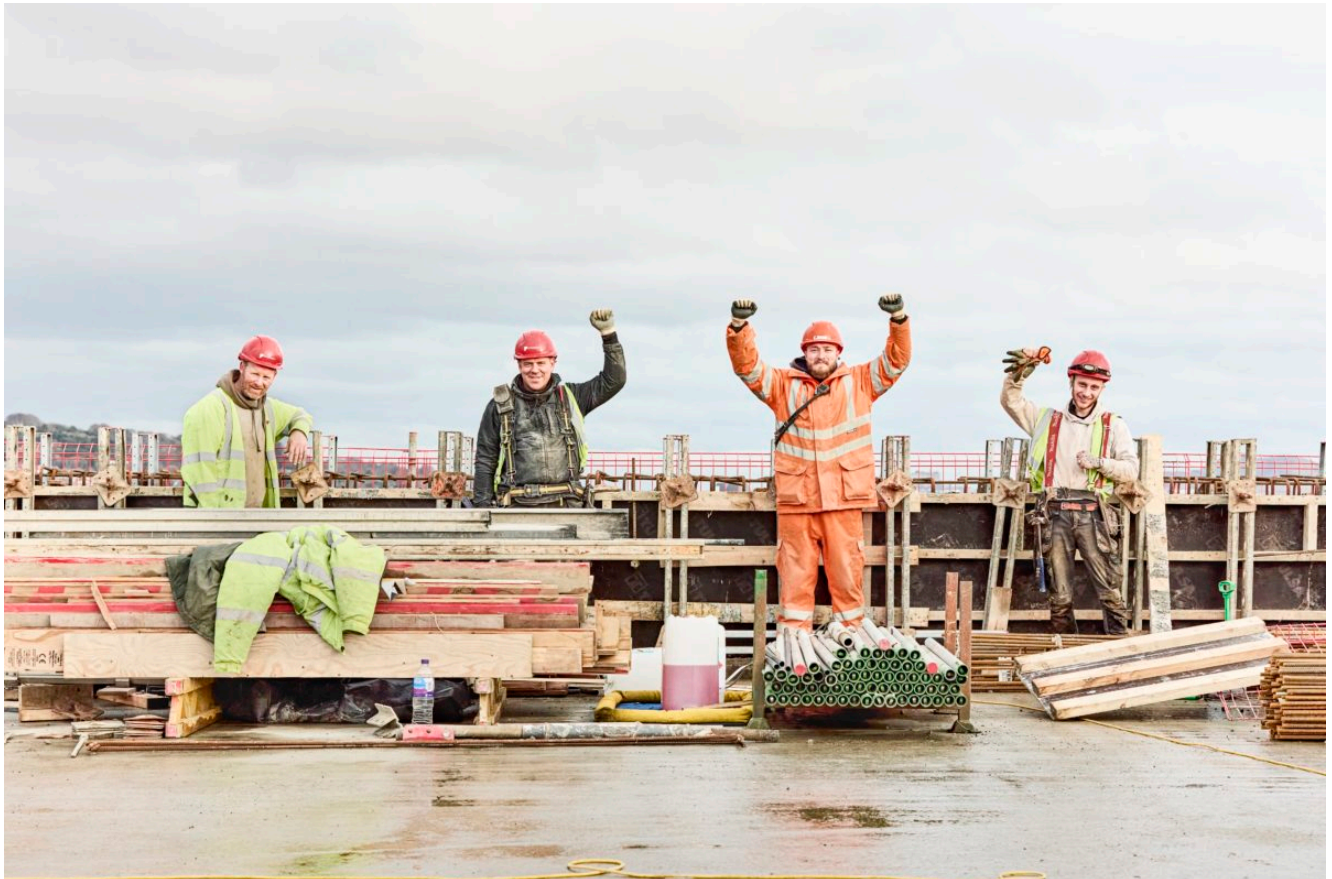
Photo of the topping out by Andy Mather
