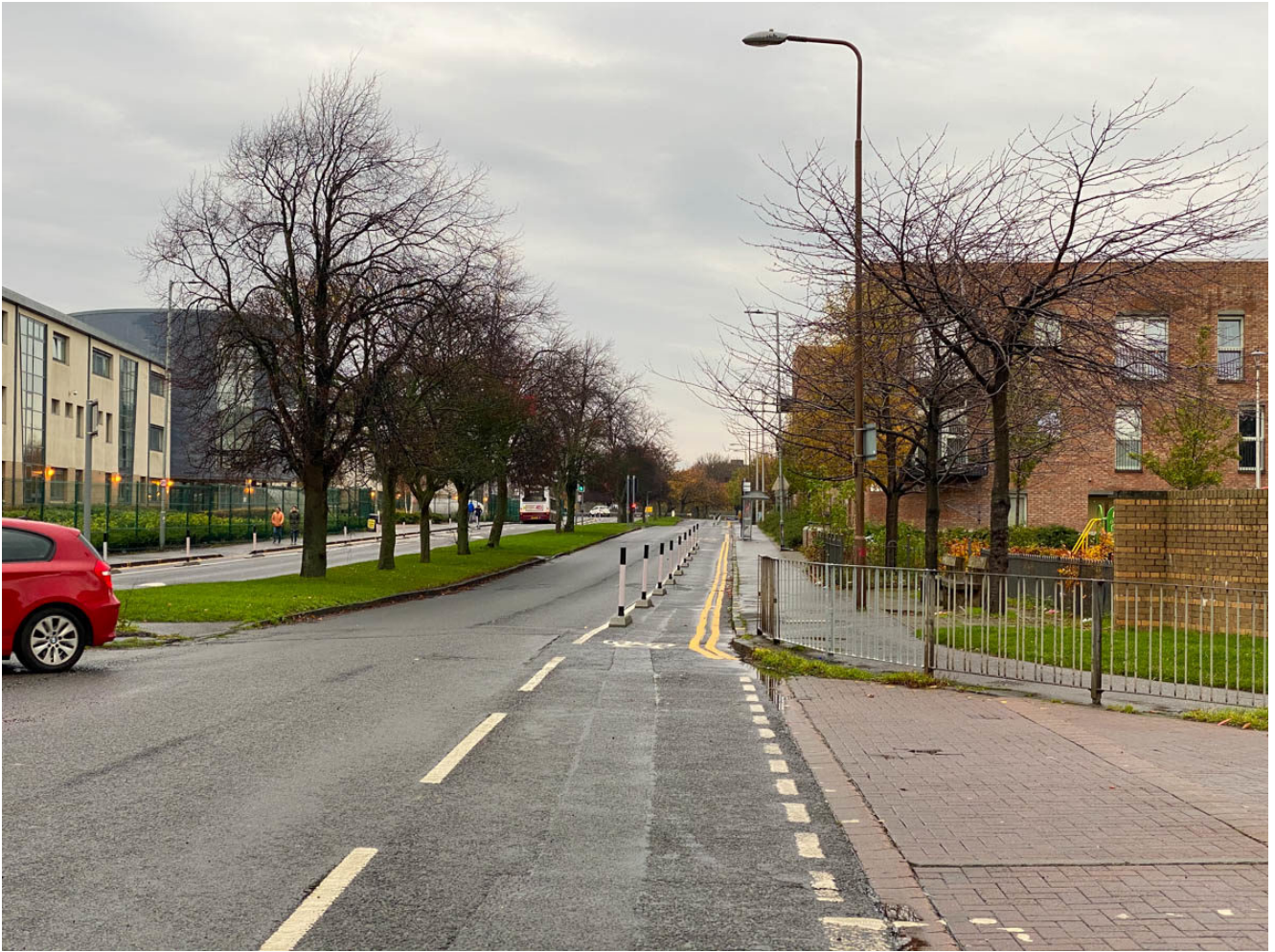
Pennywell Road where Spaces for People measures have included a new segregated cycle lane PHOTO ©2020 The Edinburgh Reporter
