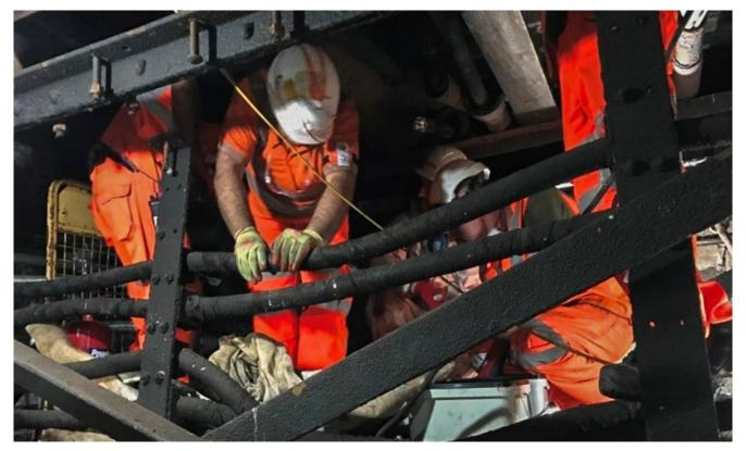
In order to access the underside of the bridge, contractors have been progressing the erection of a complex scaffolding structure – the largest since the current concrete deck was constructed in 1933 – with sections being delivered overnight from the beginning of the project to minimise disruption.
