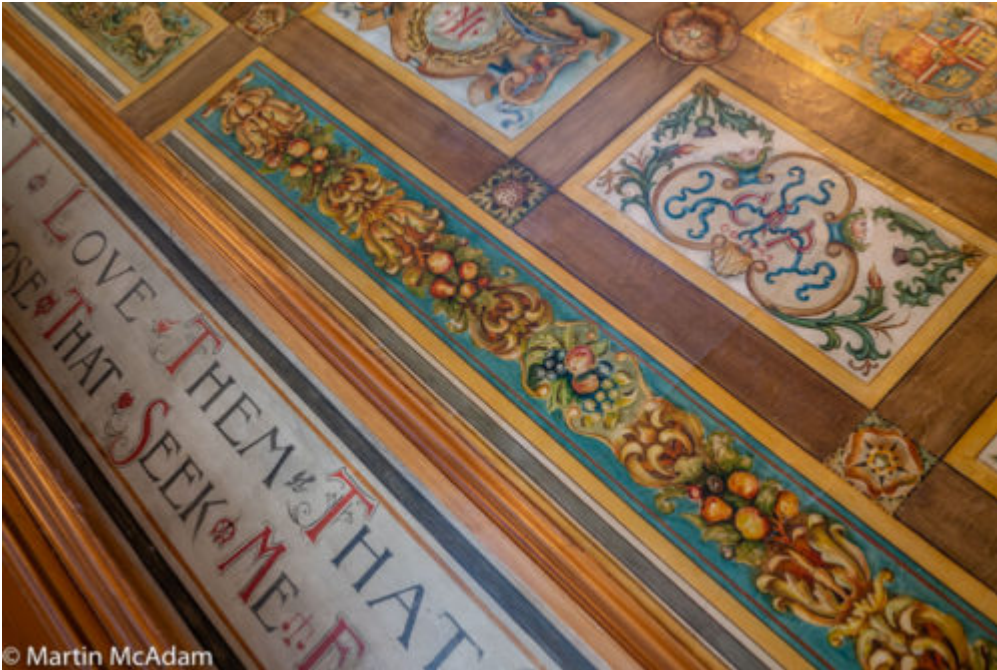
Detail of ceiling in Riddle's Court
