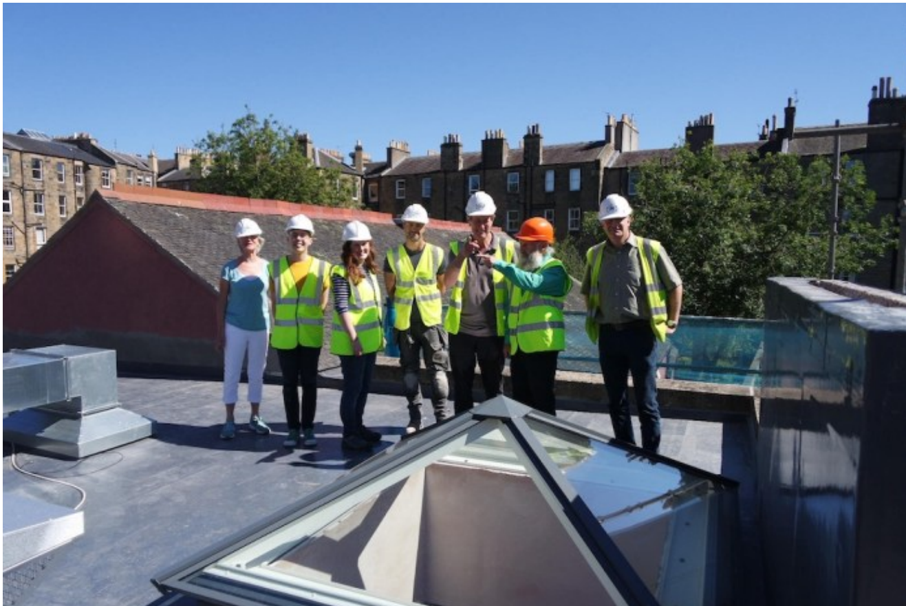
The new flat roof at St Peter's
