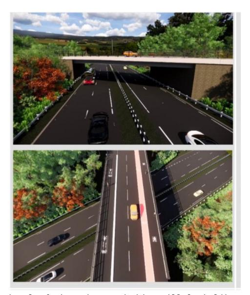
A visual of what the new bridge will look like The original bridge was built in 1964 when the Forth Road Bridge and connecting roads were constructed. The form of construction was favoured at the time but has since been found susceptible to corrosion. The old bridge deck contained a single span suspended on 'half-joints' which is no longer permitted.
