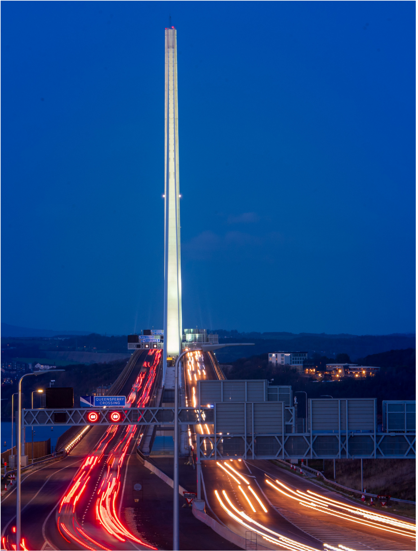
QUEENSFERRY Architectural lighting has been installed on the Queensferry Crossing, it includes uplighting for each of the main towers and strip lighting along the deck edge of the bridge. Photo Ian Georgeson
