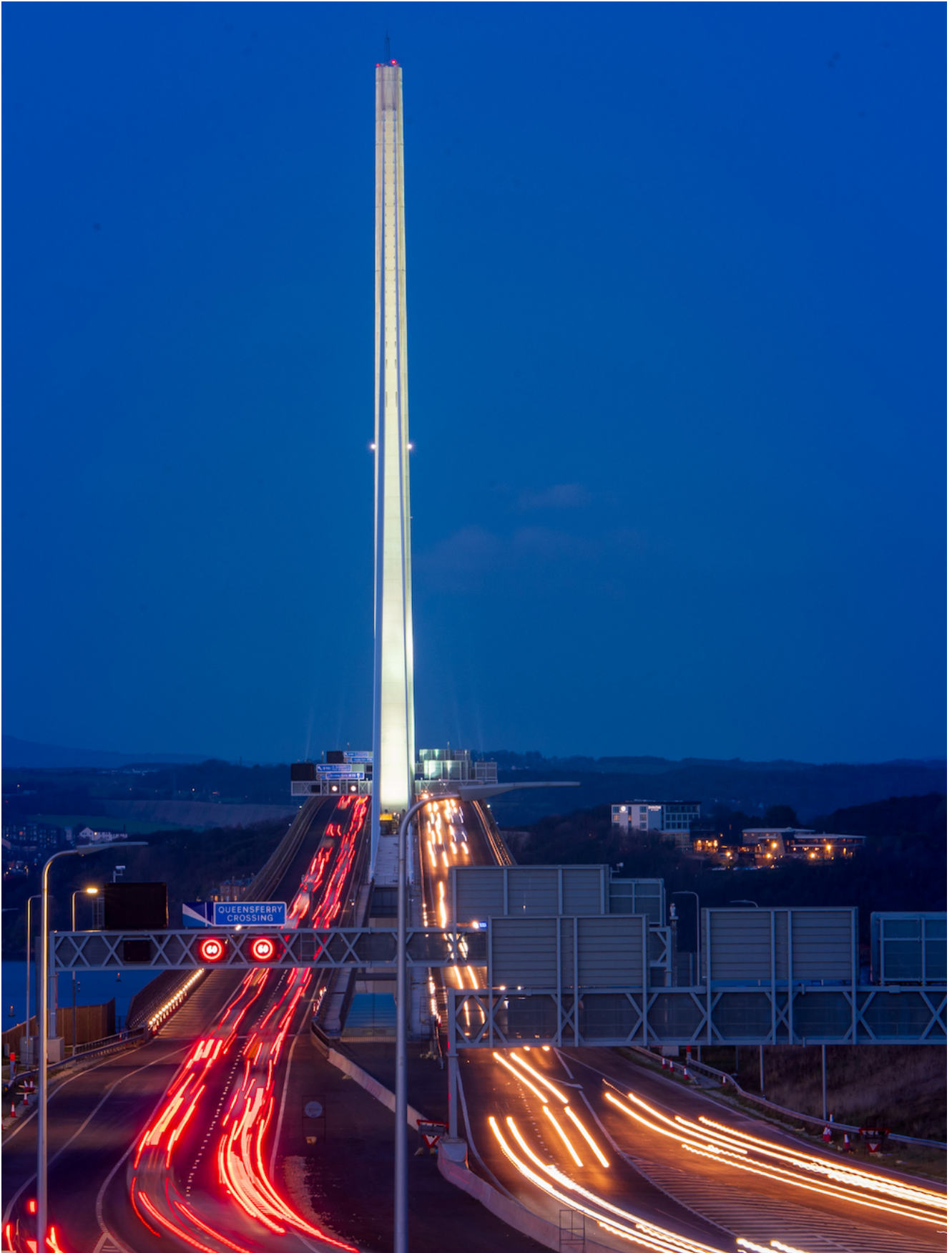
QUEENSFERRY Architectural lighting has been installed on the Queensferry Crossing, it includes uplighting for each of the main towers and strip lighting along the deck edge of the bridge. Photo Ian Georgeson
