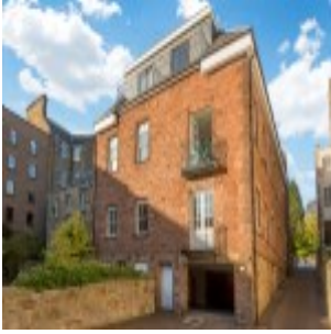
Southern elevation with balcony
