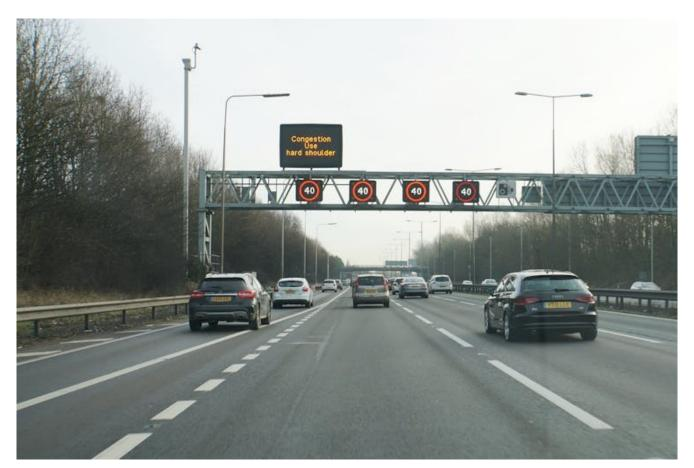
Smart motorways can reduce the speed limit to manage congestion.
