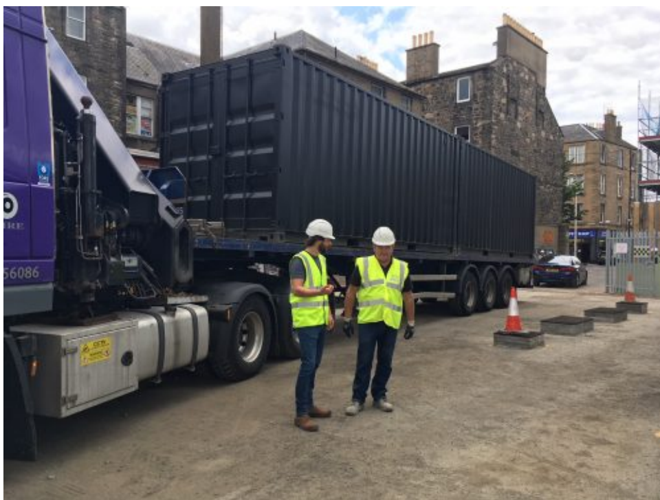
Containers arriving on the site
