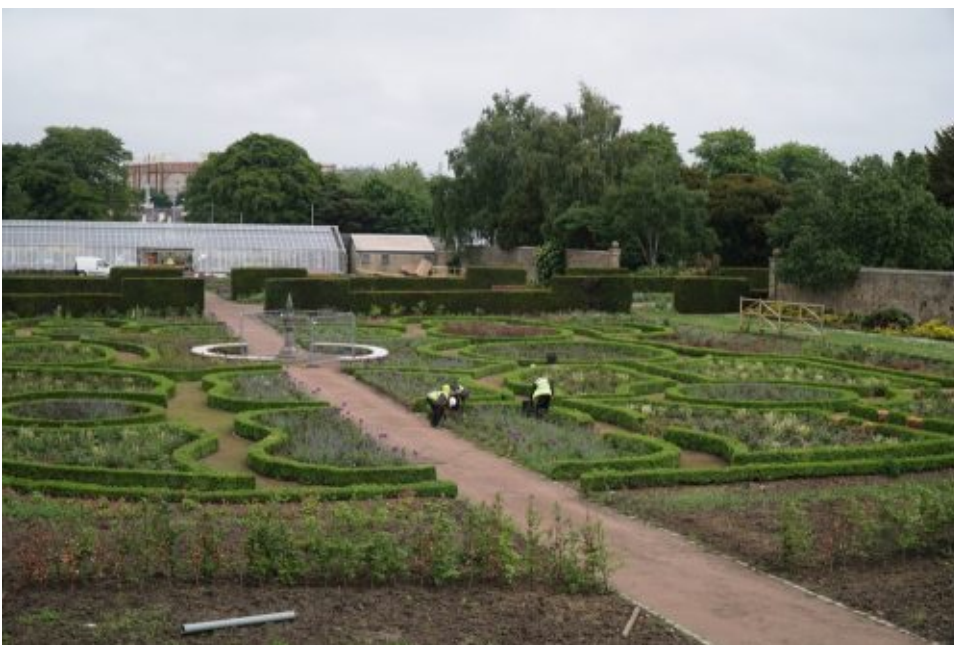
Work in progress at Saughton Park June 2018
