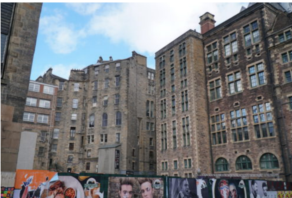
A view of the building from the Cowgate
