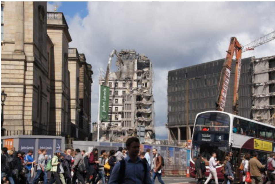
Demolition of St James Centre
