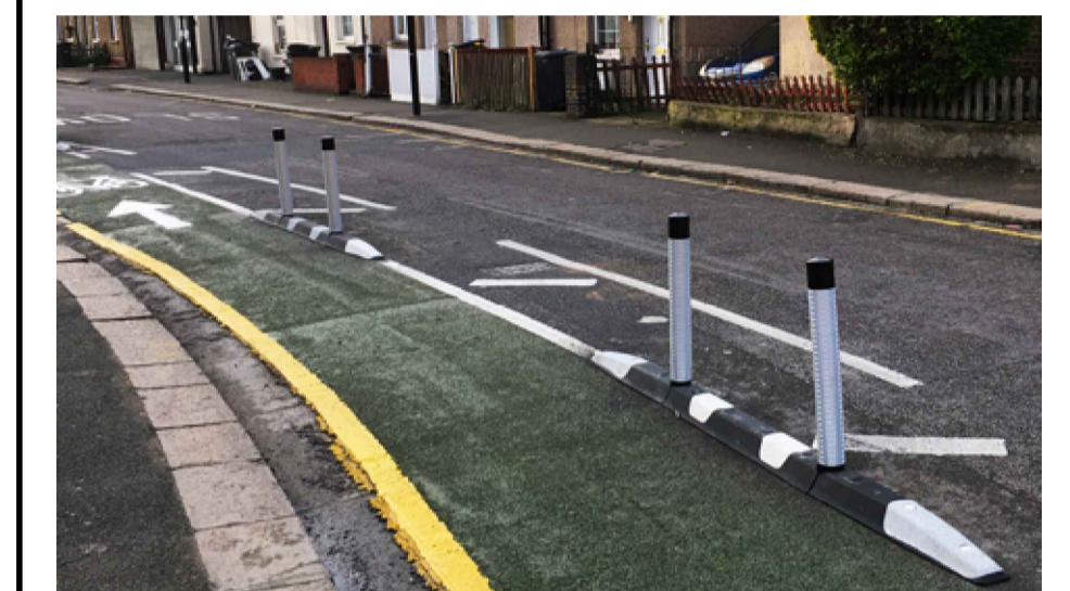
Fig 1. ORCA WAND - TO PROVIDE TRAFFIC SEGREGATION. PRODUCT 2.5m IN LENGTH & ARE BOLTED INTO CARRIAGEWAY WITH 5m GAP.
