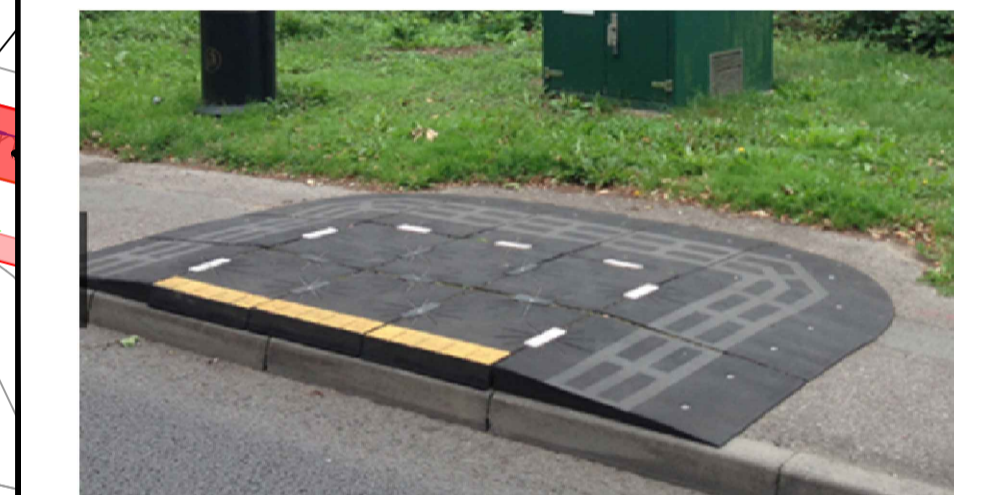
Fig 2. REDIWELED BUS PAD (OR SIMILAR)- RETAIN BUS STOPS WHERE NO LAYBY PROVIDED.
