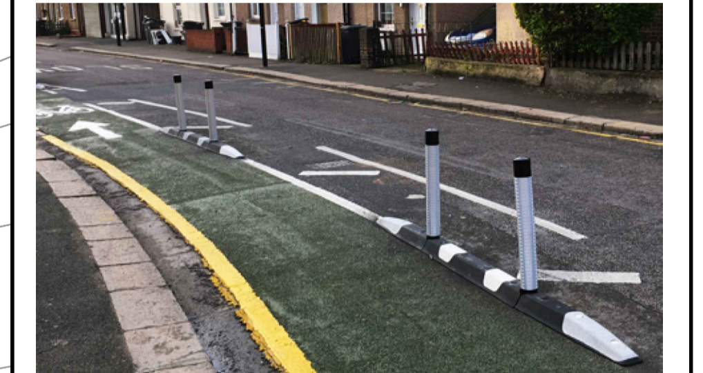
Fig 1. ORCA WAND - TO PROVIDE TRAFFIC SEGREGATION. PRODUCT 2.5m IN LENGTH & ARE BOLTED INTO CARRIAGEWAY WITH 5m GAP.
